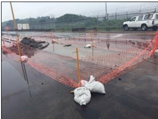
3) Construction of driveway to the HCP JV site camp – December 2019.
