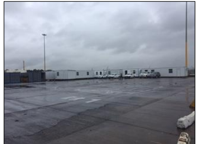
2) The establishment of the main contractor's camp- December 2019.
