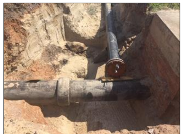
6) Laydown of pipes on site – February 2020.
