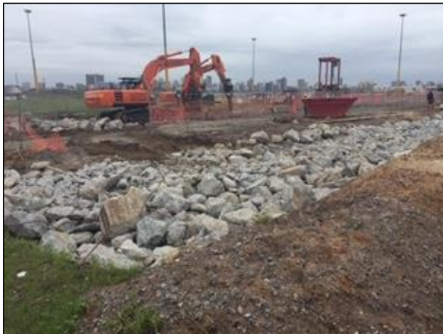
1) Laydown of pipes on site -November 2019.
