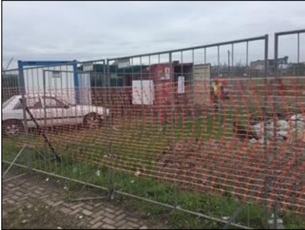
13) Establishment of Atomic Demolishers site office- November 2019.
