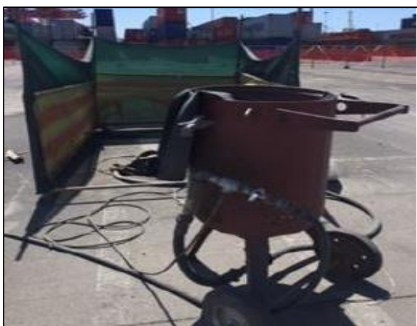
5) Sand blasting activities at the HCP JV site camp – January 2020.
