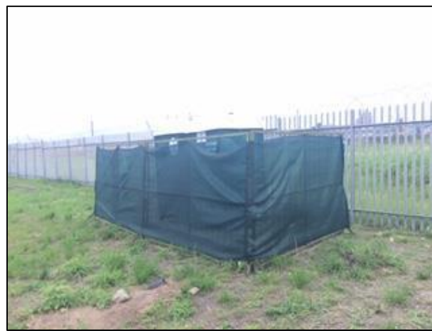
10) Provision of recycling bins on site- November 2019.
